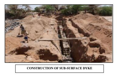
The bottom of the trench should reach the base of the productive aquifer. In case of hard rock terrain, below a limited thickness of alluvial fill, weathered zone and underlying fractured aquifer may occur. The trench should be deep enough to penetrate both highly weathered and fractured strata. In case of more open terrain in consolidated or semi-consolidated strata, the alluvial thickness may be larger and the trench should end below the alluvial fill deposit.
